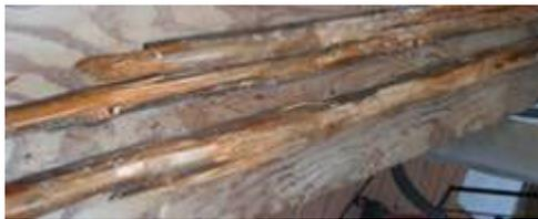
Remove any loose rot from the inside of the exterior pieces and then saturate them with CPES. These pieces will later put back in stage 3 of the restoration process. CPES can be applied with a brush like paint. The wood maintains a “wet look” for a few minutes when saturation is complete.
