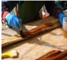
Once the cavity is treated, the new pieces that you are rebuilding the log with should also be treated. As these pieces were small brushing on CPES was the best way to do this. You will find that it soaks in a bit, however two to three coats in succession usually does it. Do NOT let it dry between coats. After you are done treating the wood let sit for a few days to completely dry.
