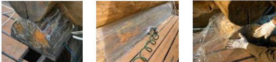
The last repair that was carried out was on a "butt end" This area exhibited a hollow sound when hit with a mallet, indicating some dry rot. For this repair, holes were drilled in to the rotten area about 4 inches apart. I used a squeeze bottle that was supplied by Coastal Epoxy Restorations to inject CPES into the area. Once again, the more the better as it slowly wicks along the wood grain and seals and helps preserves the damaged area.
