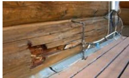
This particular home had extensive damage along one of its large base logs accompanied with some rotten corners and log ends. It was determined the deterioration was caused by two distinct issues. 1) As you can see in the above photo a water pipe drilled through the top of the log brought a lot of condensation into the log during the summer months. 2) A long and deep check or crack in the log faced up, which brought additional snow and rainwater into the log.
